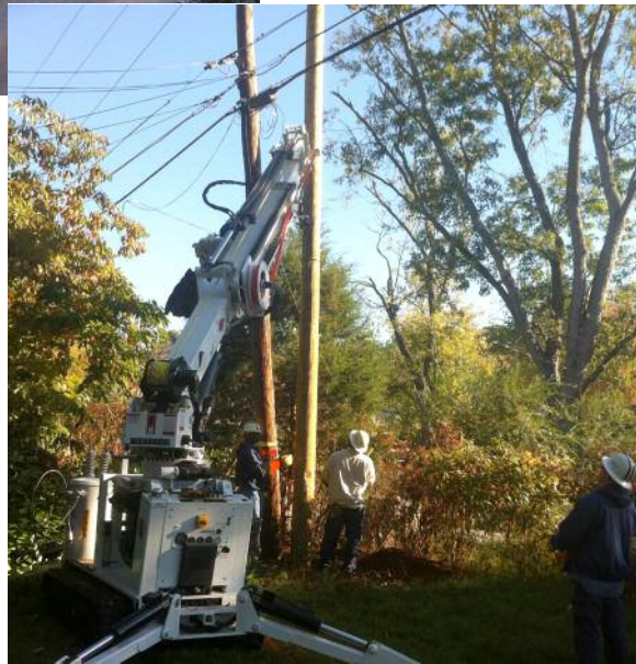
In November a backyard digger derrick was added to the Department's equipment. This will allow crews to install poles and other facilities in places where trucks cannot go. In the picture below a crew member helps guide a pole through a carport. This particular work site has electrical utilities feeding from a backyard right-of-way.
