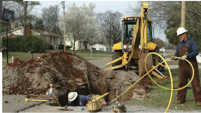
Updating the infrastructure includes replacing existing pipelines in the older sections of town. Pictured below a Gas Department crew exposes the old galvanized gas line and inserts a new yellow PE line through the pipe. At the house, another crew member fits the galvanized pipe holding the PE line with new fittings and resets the meter.
