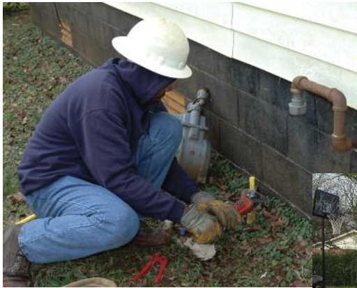
Updating the infrastructure includes replacing existing pipelines in the older sections of town. Pictured below a Gas Department crew exposes the old galvanized gas line and inserts a new yellow PE line through the pipe. At the house, another crew member fits the galvanized pipe holding the PE line with new fittings and resets the meter.
