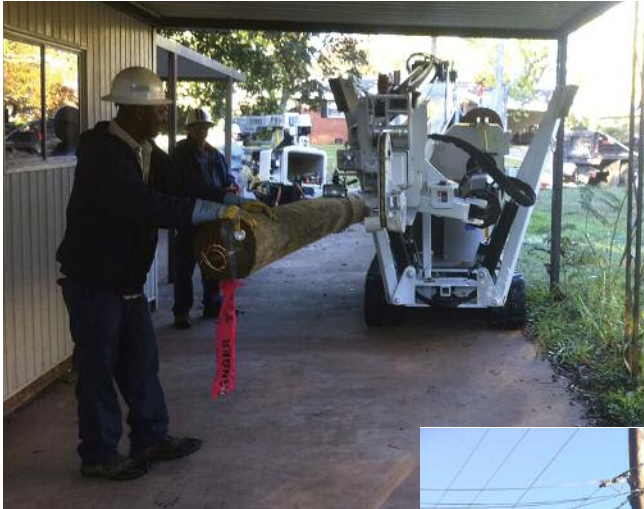
In November a backyard digger derrick was added to the Department's equipment. This will allow crews to install poles and other facilities in places where trucks cannot go. In the picture below a crew member helps guide a pole through a carport. This particular work site has electrical utilities feeding from a backyard right-of-way.
